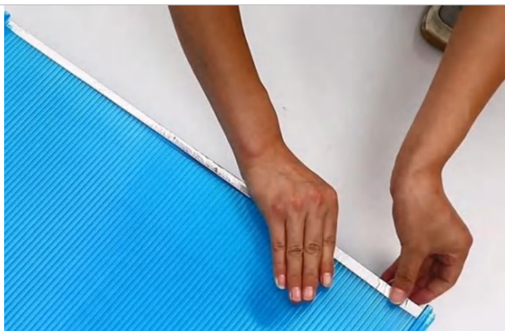
2. Stick aluminum tape/breathable tape on both ends, remove the bottom film of the board
