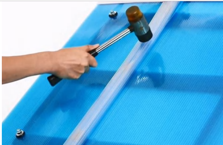
8. Install the pressure strip to connect the two boards
