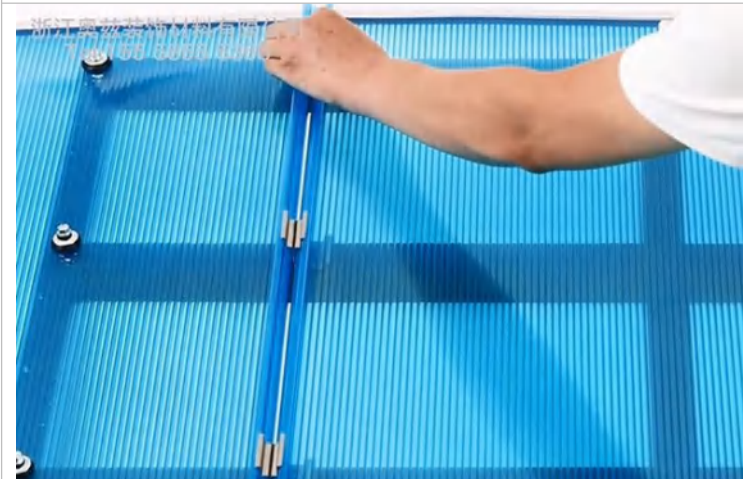
7. Install the second board
